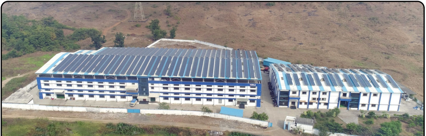
Unit - 1: Heat Shrink Tube, Moulded Shape, Cable Accessories and PVC Moulding Factories - Palghar
