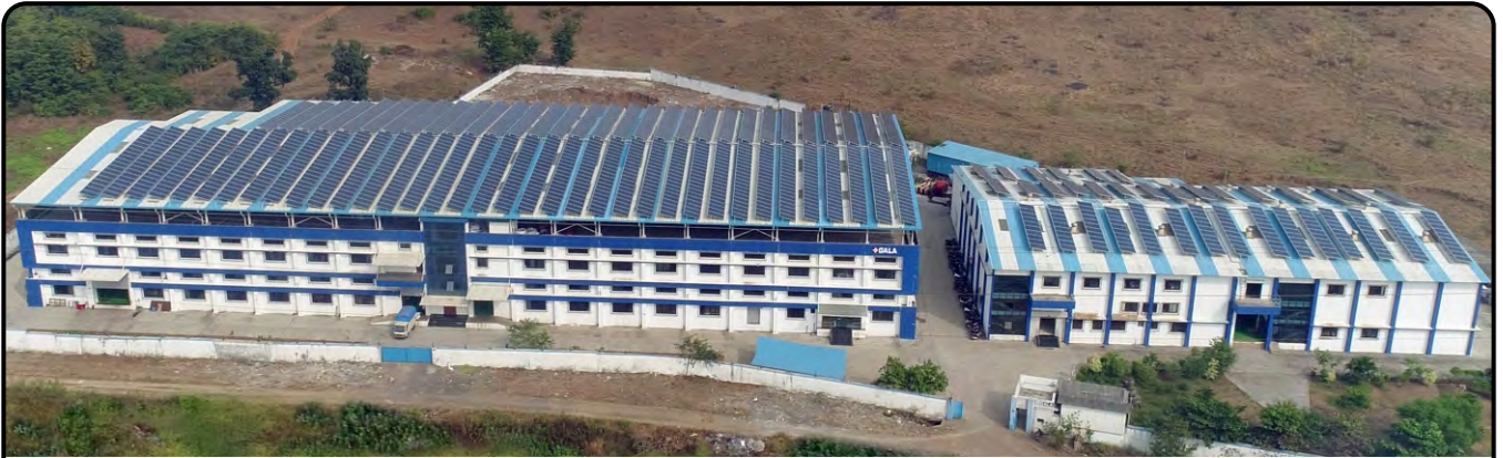
Unit 1 : Heat Shrink Tube, Moulded Shape, Cable Accessories and PVC Moulding Factories - Palghar
