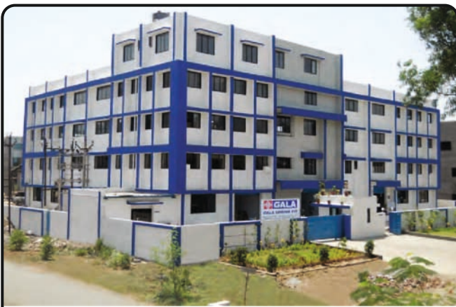
UNIT - 2 Moulded Shapes Factory - Surat (100% EOU)
